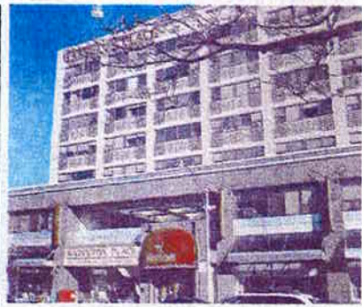
Right, Tapestry at Village Gate West, under construction. Above, Hazelton Place in busy Yorkville. DARC Y MCGOVERN/THE GLOBE AND MAIL
